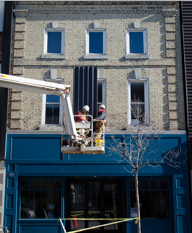
Two workers use a crane-lift to bring siding up to the top of a heritage building in downtown Belleville.
